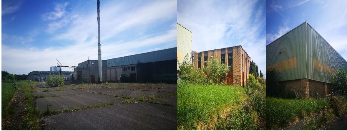
FIGURE 2.4 VIEW OF THE EXTERIOR OF THE EXISTING BUILDINGS WITHIN THE SITE
