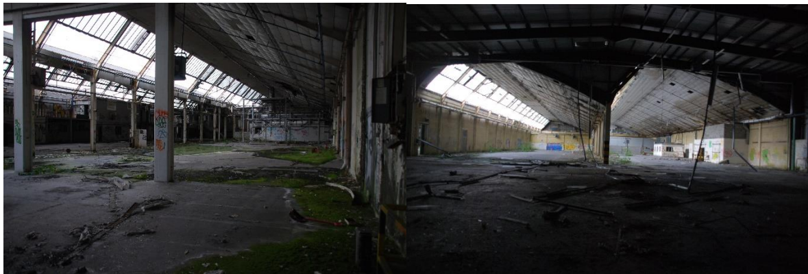
FIGURE 2.5 VIEW OF THE INTERIOR OF THE EXISTING BUILDINGS WITHIN THE SITE
